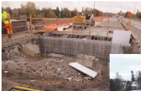
Madawaska River Bridge Arnprior
